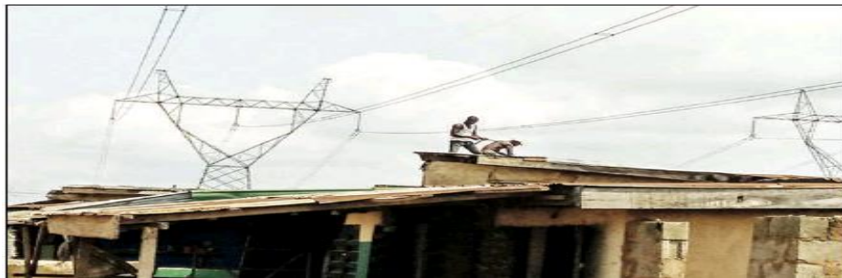
Figure 1.1: Building directly under high-tension wire at Ore, Ondo State.
