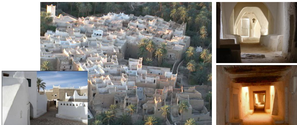
Figure 4: The Organic compact urban fabric for Ghadames City, Libya (Left) – The shaded arcaded alleys with openings for lighting and ventilation (right) [5]
